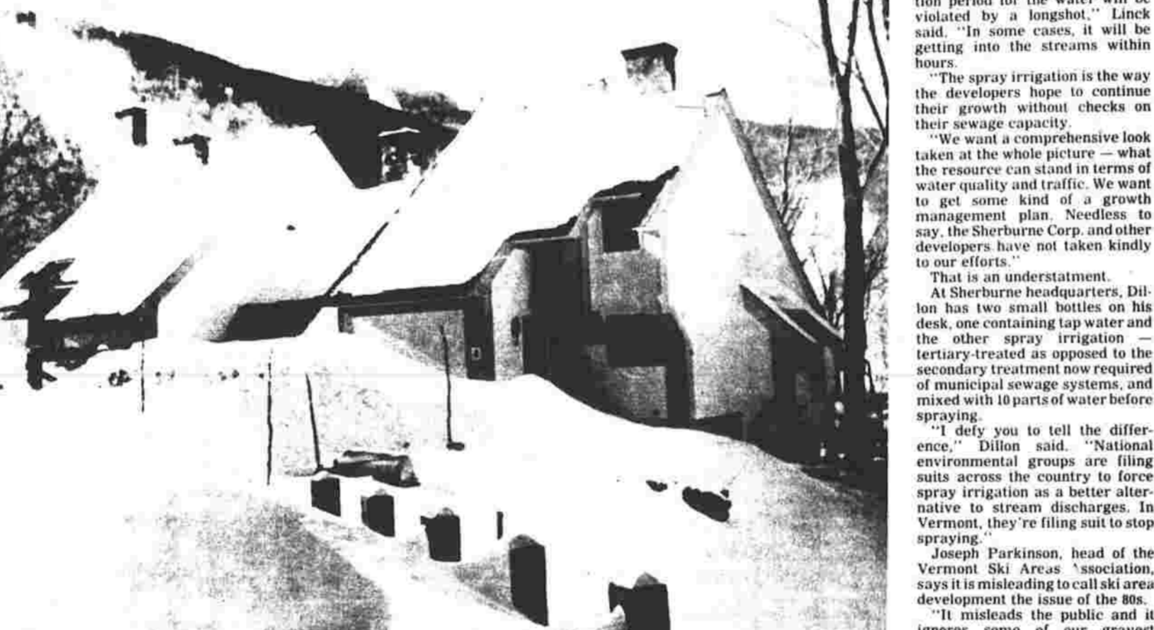
Northern New Englanders find themselves in the midst of a tax shelter boom. Condominiums such as this one in Killington, Vt., are creeping onto mountainsides and nesting along the two-lane highways that snake through scenic river valleys in Vermont, New Hampshire and Maine.
